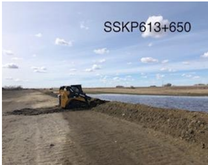
Skid steer used to create a break in roach line to alleviate the water to dry quicker
