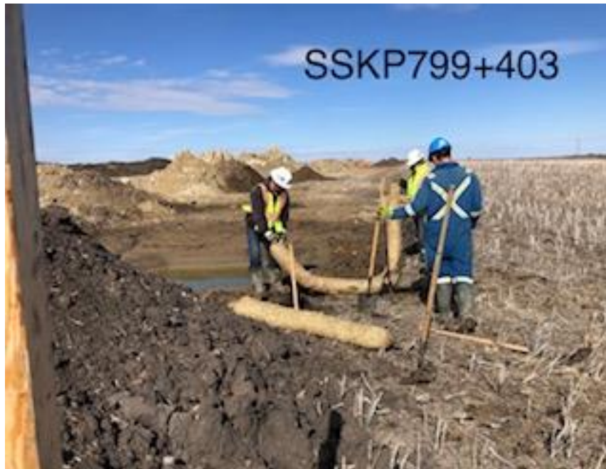
Erosion control devices – straw wattle being installed
